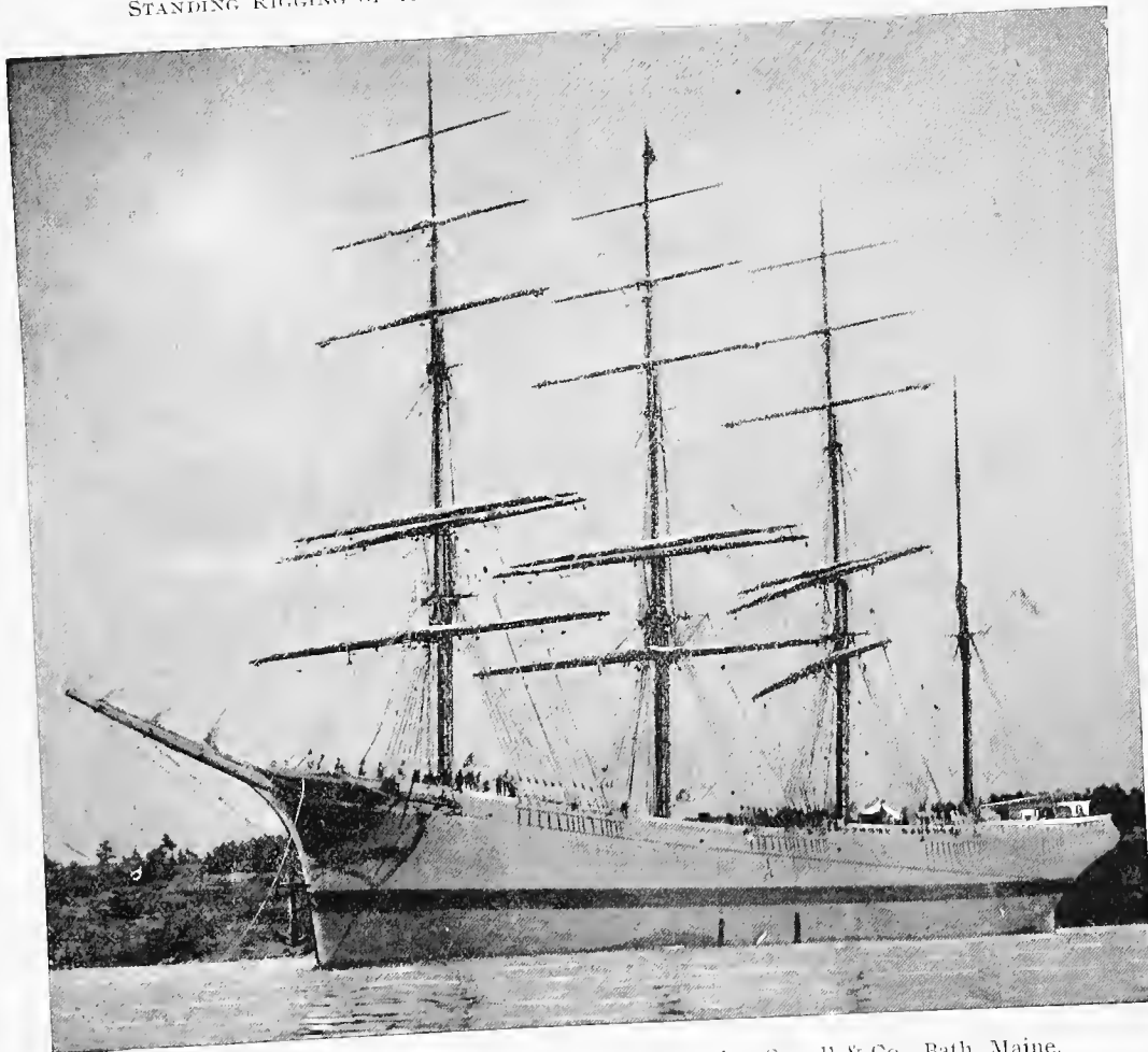
STANDING RIGGING OF THE ROANOKE, SHOWING THE IRON TURN-BUCKLES.
